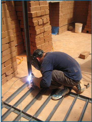
Jason welding up the water tower
