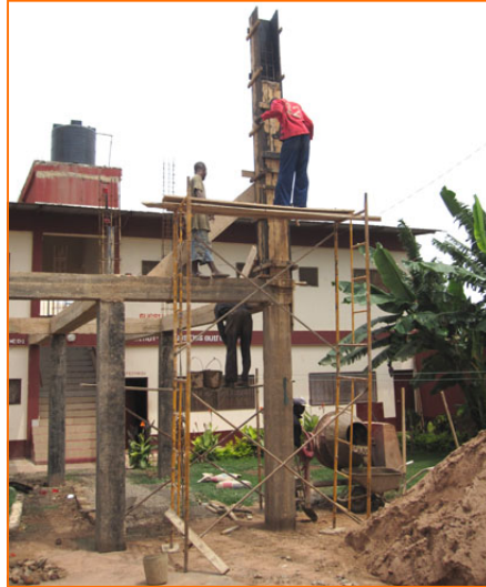
Pouring the second story columns of the solar panel support structure
