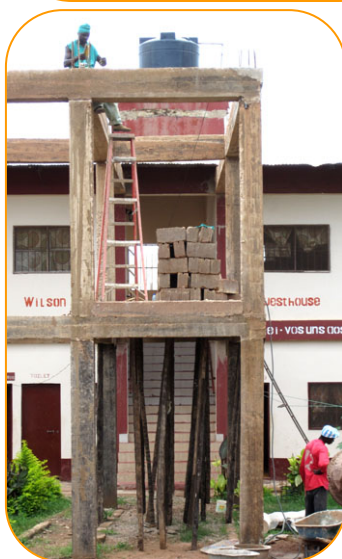
Building a secure room off the ground using the pillars of the solar support structure
