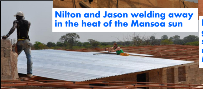
Our friend from New Zealand, Aidy, attaching the corrugated zinc to the steel frame
