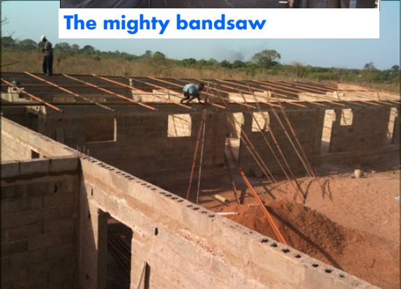
Setting the frame for the roof on the L-shaped dorm
