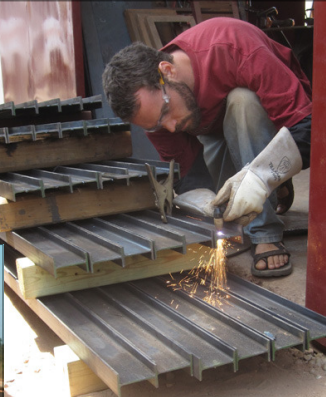
Slicing through roof girders with a plasma cutter
