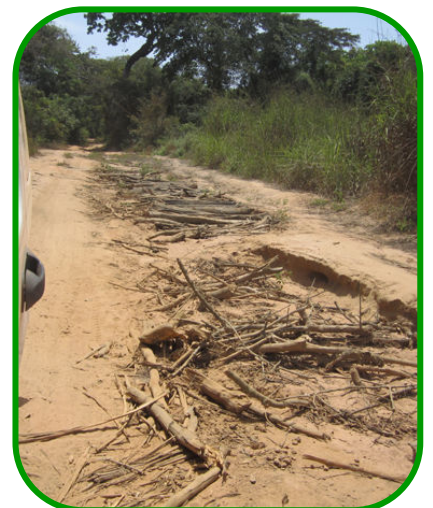
To keep a road from washing out in the rainy season, just cover it with heavy logs
