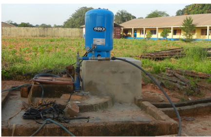
The new water pump and blue pressure tank installed next to the well at WAVS vocational school
