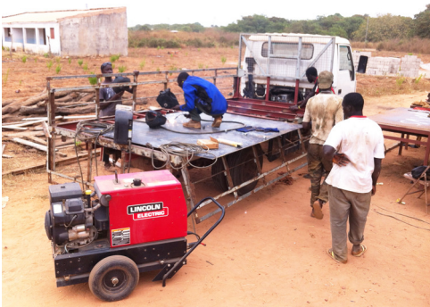
Making a new bed for the school's truck - scrap yard steel underneath and new diamond plate on top
