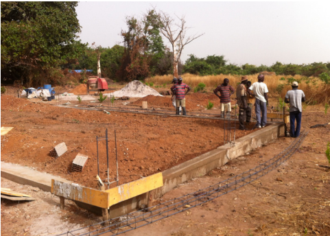
The construction crew working on the foundation for the drinking water filter factory
