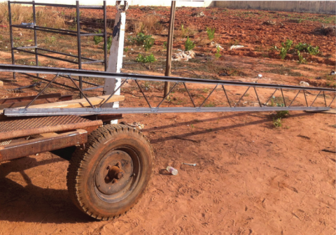
One of the roof trusses for the drinking water filter factory
