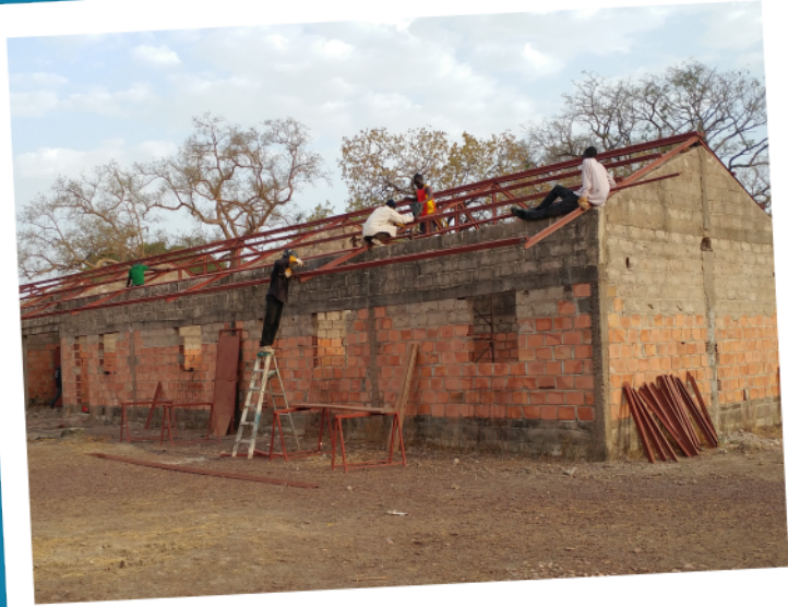
Purlins being set. Almost ready for sheet metal.
