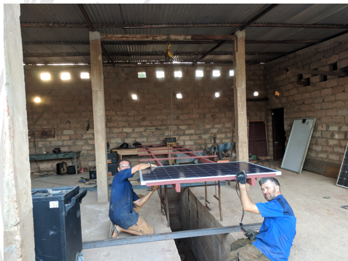
Américo and I fastening the solar panels to the metal frame we welded on-site.
