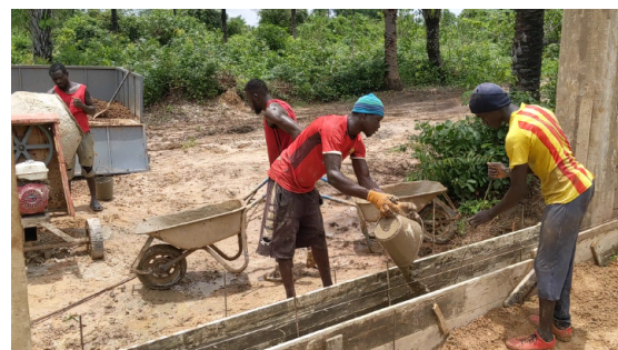
Pouring the gate support beam with a piece of spine-up angle iron for the wheels to roll on.
