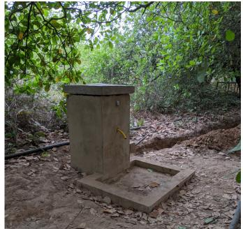
I was able to leave with the tap fully functional, though it's lacking its finishing. Once we're sure it doesn't develop any leaks, the lid will be leveled and sealed, the structure will be painted, and the bottom of the catch pan tiled.
