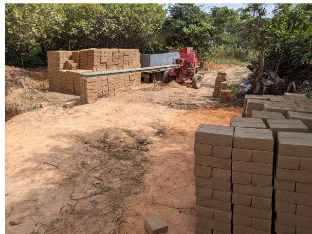
Blocks are piling up! The team has produced more than 4,000 in the last couple of weeks! (They're 6" x 12" and 4" tall, for scale.)
