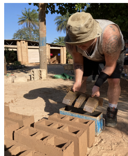
They also made several batches of compressed adobe and cinder blocks!
