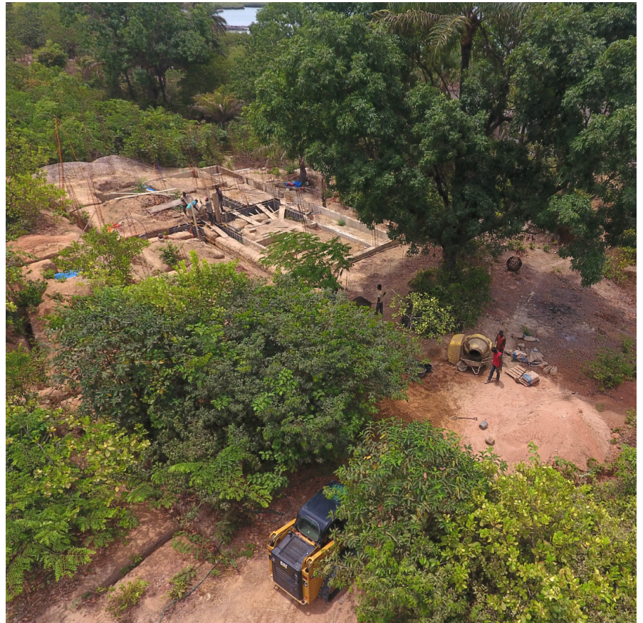
The tractor is helping speed up our cement-mixing station under the tree by keeping supplies at the ready! From there the concrete is taken by wheelbarrow to the pour.
