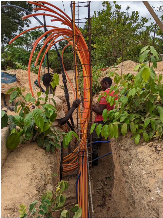
Plastic conduit for the eventual house electrical installation is being wrangled/organized in preparation for being poured into the foundation wall.
