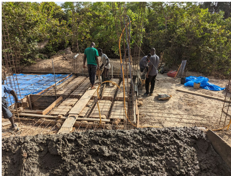
In other cases, we needed to finish work that was in process but would be damaged by the rain, like pouring the ceiling of the one-room basement in our house whose formwork was already in place but susceptible to rain damage if left unpoured.
