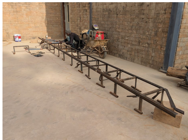
Benildo is at the far end laying out the truss pieces to prepare for welding.
