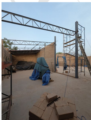
After the last steel column of this side of the shop was set, the welders and masons had a friendly race. The masons built the last section of wall while the welders set the roof
